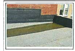
PHOTOS: ROOF AREA 5
