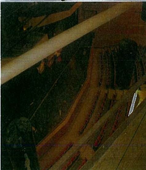
Picture 1- View of Railing
