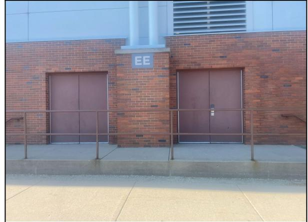
The aluminum doors are typically part of an overall glazing system and are used in places to provide architectural detail, primarily at the main entrances. Hollow metal doors are usually found at utility entrances and doors going into specific building areas, such as music rooms, gymnasiums, natatoriums, fieldhouses, scene shops, automotive classrooms, etc.
